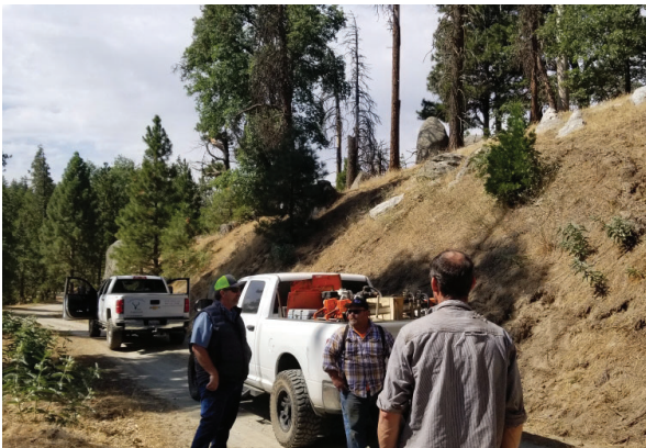
Meeting on roadside project site
